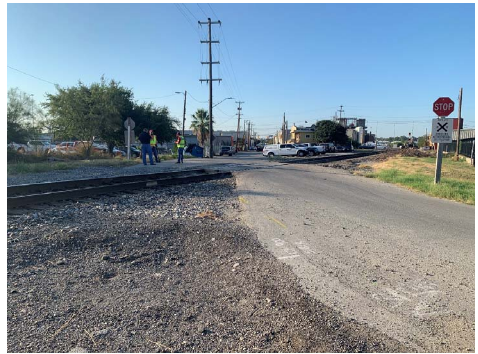
S San Marcos - 42" RCP to be Grouted (Upstream to Downstream Structure)
